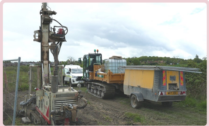
Ground investigation works on the Puddlebank
